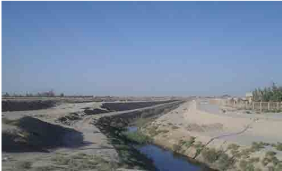
Fig. 1. Drainage Project of Sistan Plain (source: regional water corporation of Sistan and Balouchestan, 2014).
